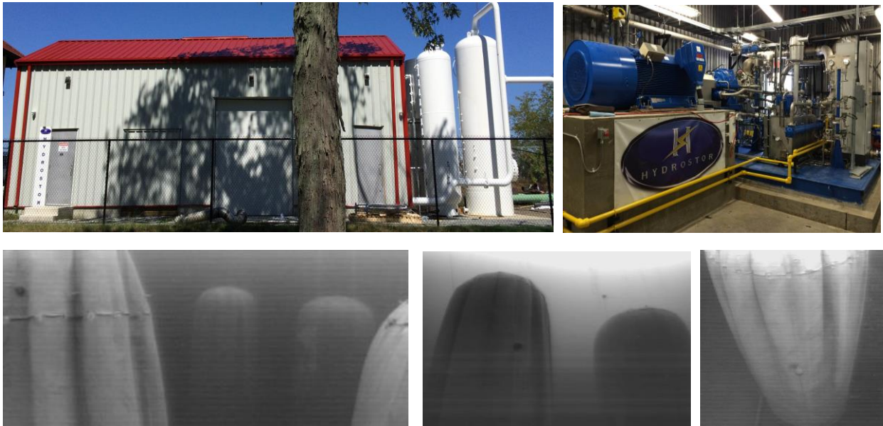
Photos: building – upper left; machinery – upper right; underwater air storage system – bottom row
